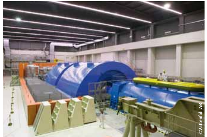
Turbine hall in nuclear power plant
