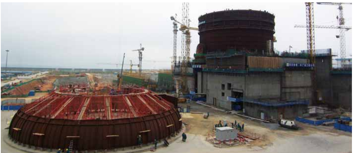
Nuclear power plant under construction
